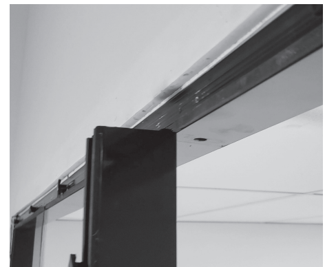
IV.15. Gently bend vertical profile to expose the \frac{1}{2} fastener hole and fasten the horizontal profile to the ceiling using fasteners of your choice.
