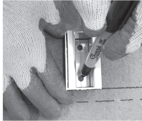
IV.10. Using F10 Floor Bracket Setup mark screw location.
