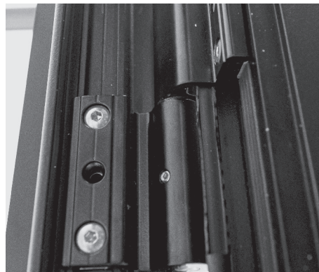
V.4. Check the level one more time and fasten the jamb to aluminum profile using S10 Screws .
