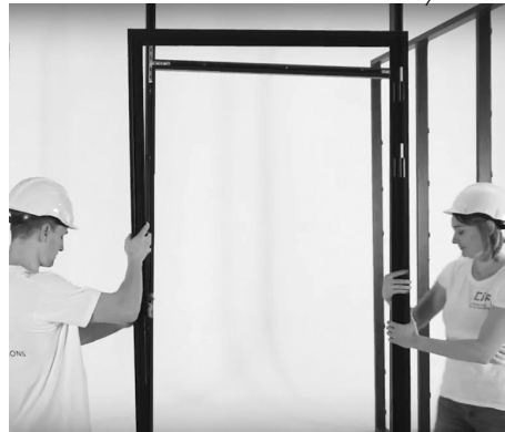
V.2. Install the Jamb into the opening and make sure it fits correctly and is level. Pull back the jamb few inches and remove blue protective strip from the door seal. Once the strip is off apply pressure to set the jamb in place. Make sure it is level.
