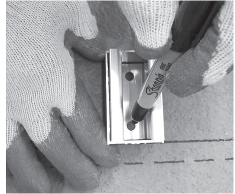
IV.11. Using F10 Floor Bracket Setup mark screw location.
