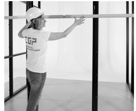
V.2. Install the Jamb into the opening and make sure it fits correctly and is level. Pull back the jamb few inches and remove blue protective strip from the door seal. Once the strip is off apply pressure to set the jamb in place. Make sure it is level.
