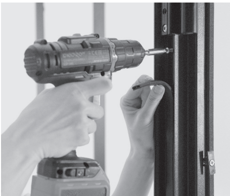
V.3. Remove black rubber gasket from the inside of the door jamb.
